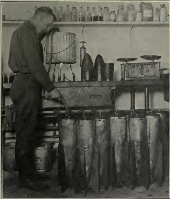
FIG. 110.—Loading Bombs with “Solid” Oil.
